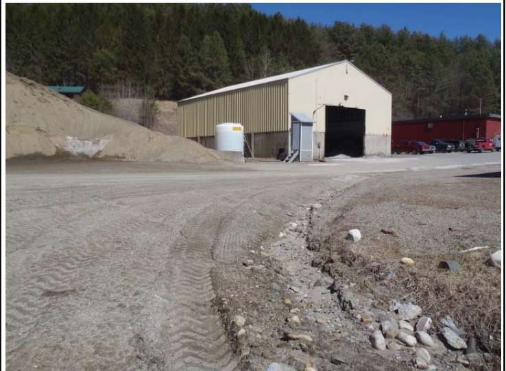
Photo 2. Visible “creep” of the sand storage pile
