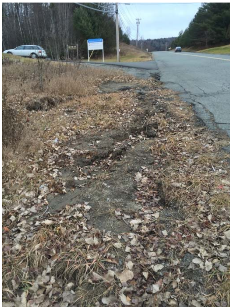
Photo 1: Erosion along the road shoulder
